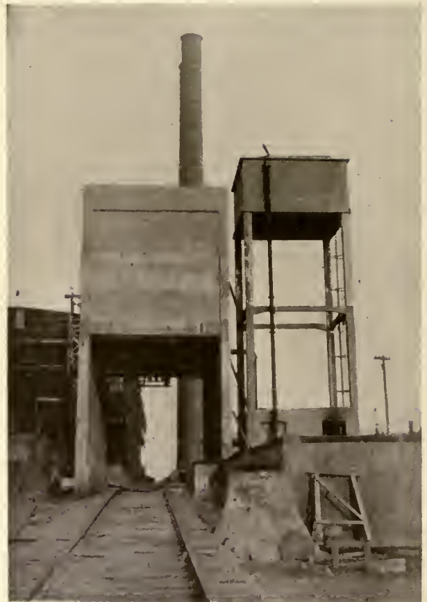
COKE QUENCHING PLANT
